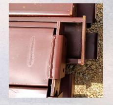
Structural steel has a painted finish typically in the red although can come in many colors. The paint is intended only to protect the steel during construction and transport and is easily damaged.
