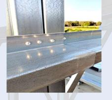
On site COLD FORMED main frame is typically both bolted and screwed together using pre-drilled plates. COLD FORMED buildings can require some cutting/coping and drilling of braces on site.
