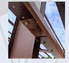
On site a Structural Steel main frame is typically bolted together with plates already welded in place in the factory. Structural Steel buildings can require some welding and drilling on site.
